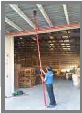
Checking of Smoke Detector
