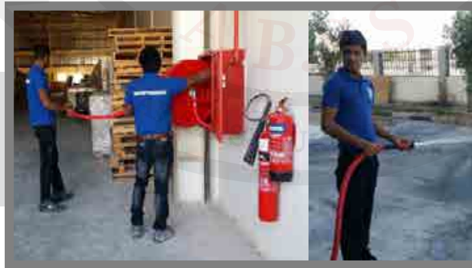
Flushing of Water using Fire Hose Reel (checking and maintenance)
