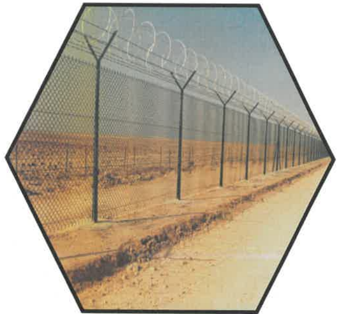
Chain Link Fence IN RILC
