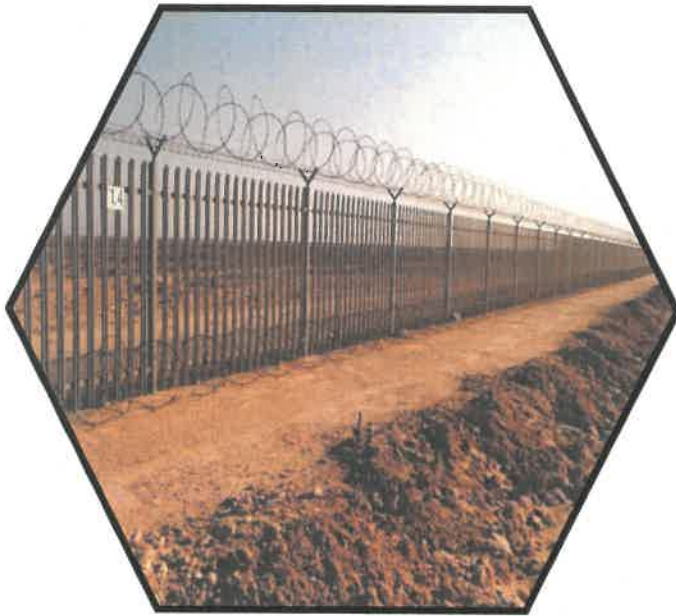
Palisade Fence IN RILC
