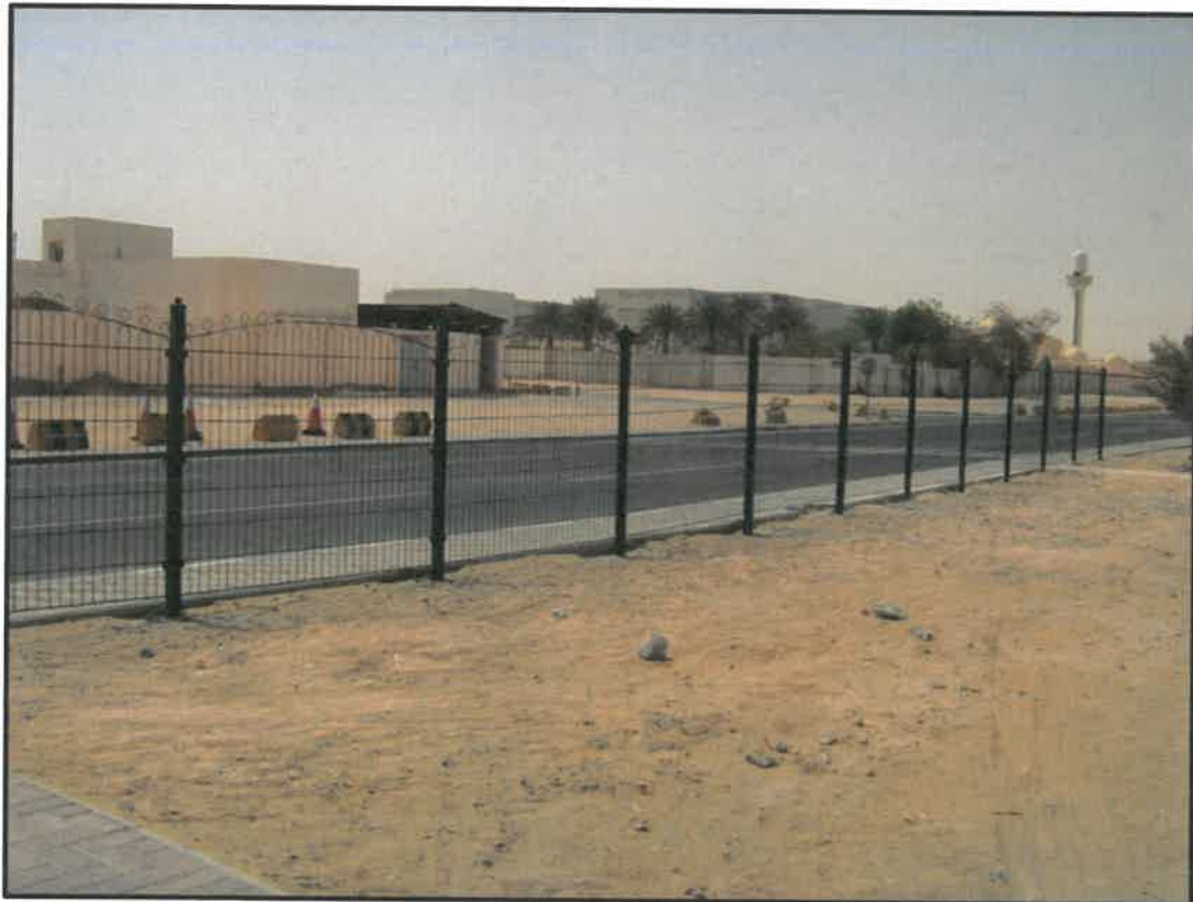
Pedestrian Fencing in Al Luqta (Near Al Luqta Gymnasium Hall)
