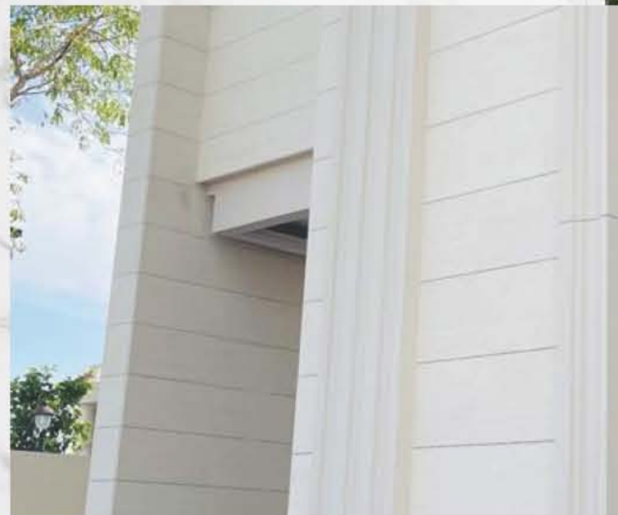
Stone Mechanical Cladding - Ventilated Facade
