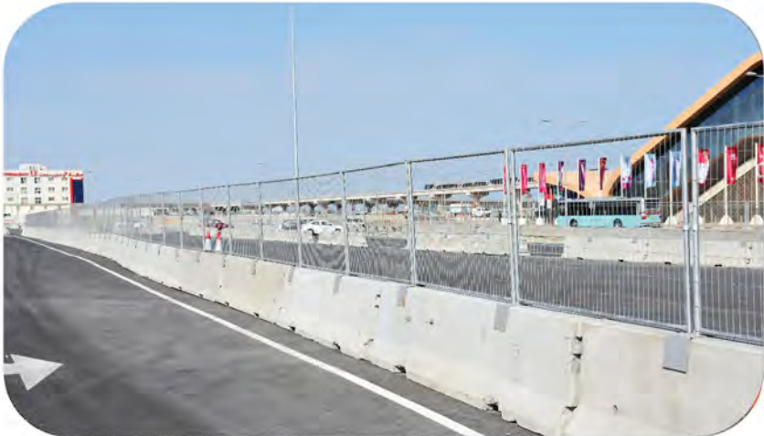
Temporary Fence Above Concrete Barrier
