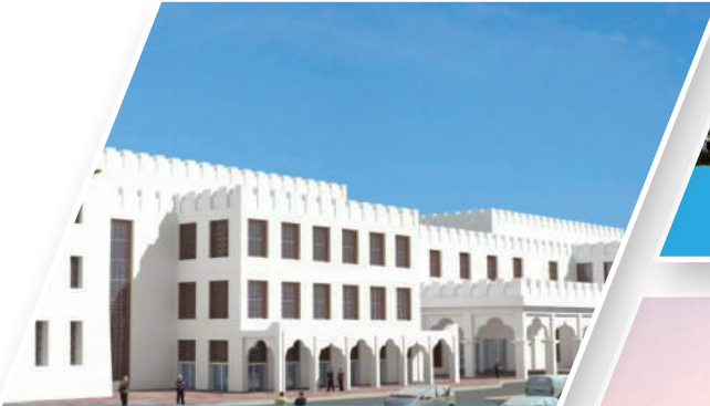
WORKERS' HOSPITAL AT RAS LAFFAN
