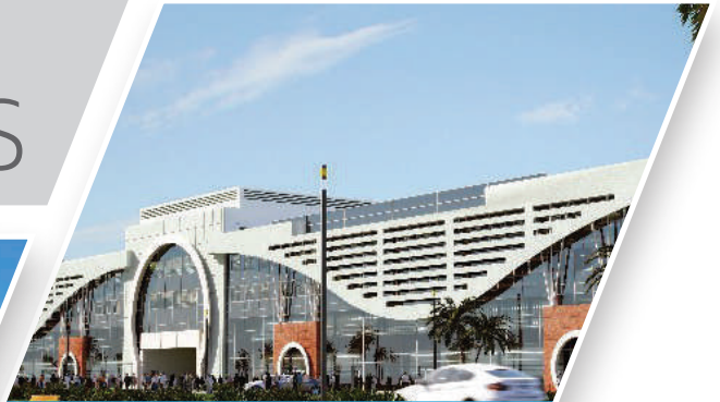
BARWA COMMERCIAL AVENUE
