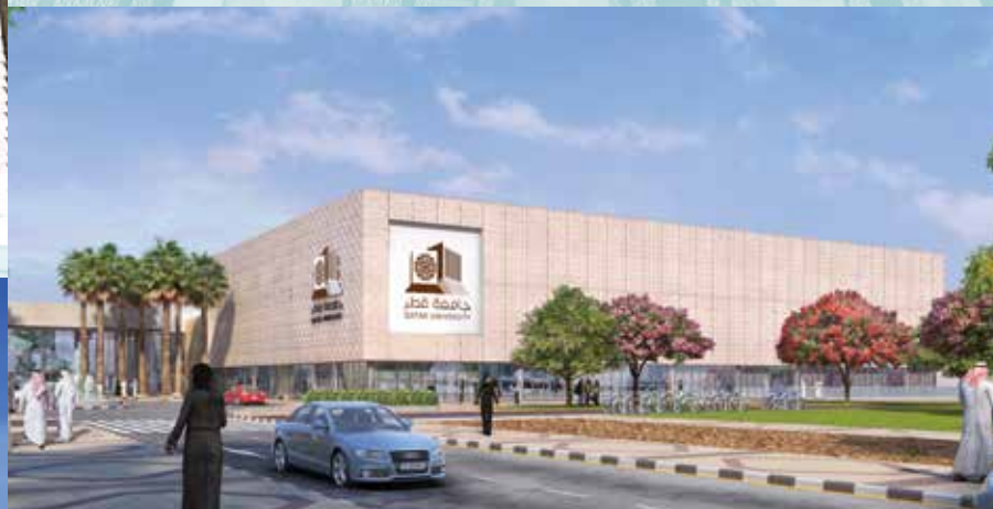
Qatar University- Sports & Utility Complex Curtain Wall
