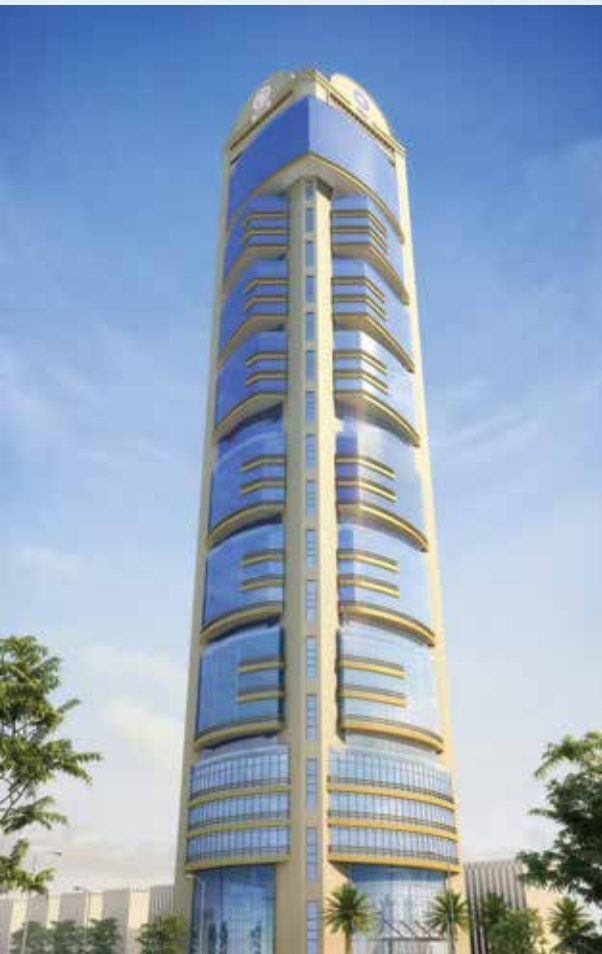
Seeliya Tower Curtain Wall
