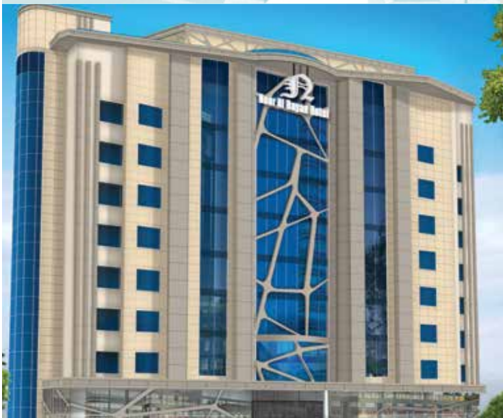
Noor Al Bayan Hotel Curtain Wall 1,605 Sqm.
