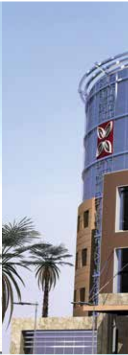
Hilton Garden Hotel Curtain Wall
