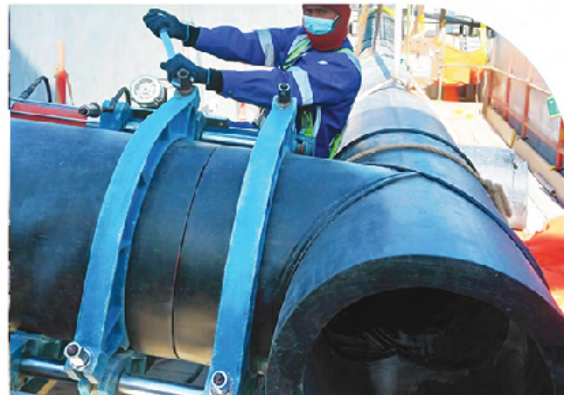
Project - Airport Area - Hdpe welding works
