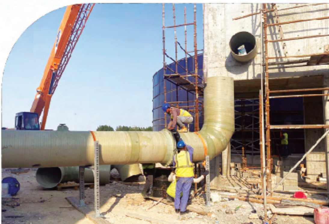
Project - Baldna Farm - GRP Lamination works
