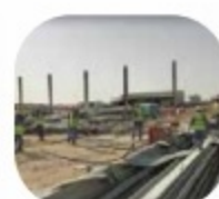
HV & LV CABLE LAYING, JOINTING AND TERMINATIONS
