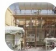
ERECTION OF 800MVA POWER TRANSFORMER
