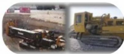
CABLE TRENCHES AND HDD DRILLS
