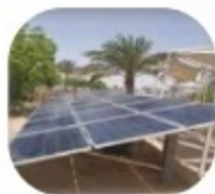
EPIC OF SOLAR PANEL MAINTENANCE
