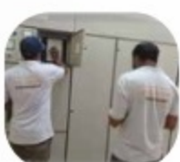
SMART METER INSTALLATION
