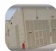
SUBSTATION AND RESIDENTIAL CIVIL WORKS
